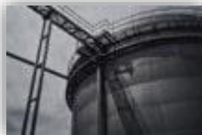
Refineries, chemicals plants
